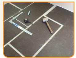
If necessary, use a straight edge, level or equivalent to ensure back edges are even. Use a hand roller, rubber mallet to roll or tap and firmly secure the end seams. End seams should be
