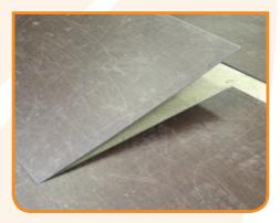
Install the next tile adjacent to the first tile by holding the tile at a 30 angle and dropping the female/groove side of the tile into the male/tongue side of the first tile, ensuring edges are aligned.
